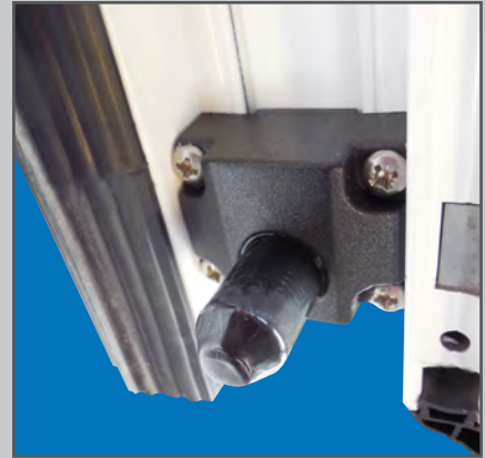
Retained roller guides
