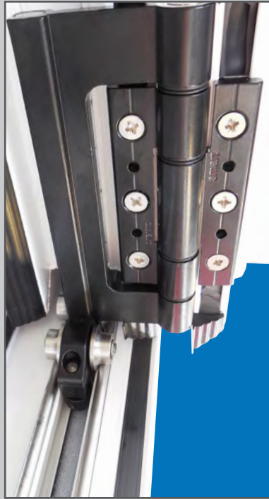
View of retained roller hinge
